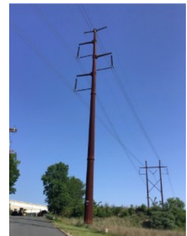
Example of a weathered Steel structure
