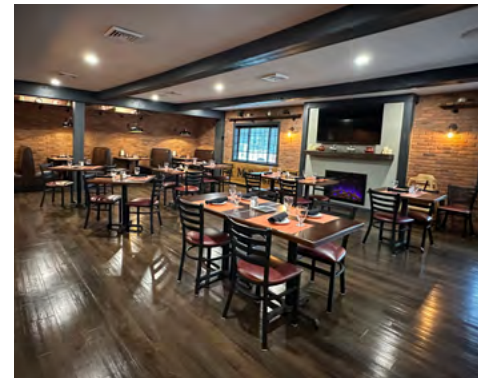
LED lighting and heat pumps installed at McSwiggan's Pub and Restaurant not only delivered energy efficiency, but also a comfortable and inviting interior.
