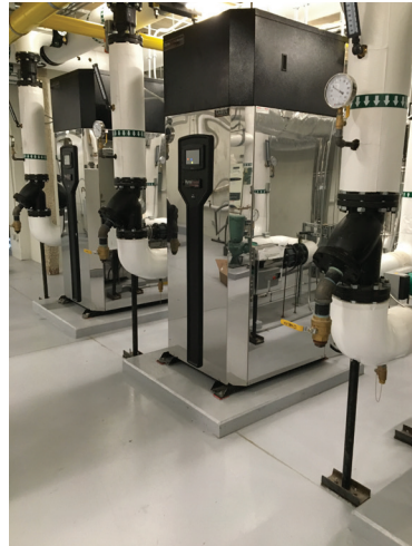
New Central Heating Plant
