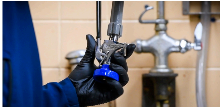
High-efficiency pre-rinse spray valves installed in commercial kitchens provide a consistent spray pattern, clean a larger surface area and are engineered to last and avoid leakage.
