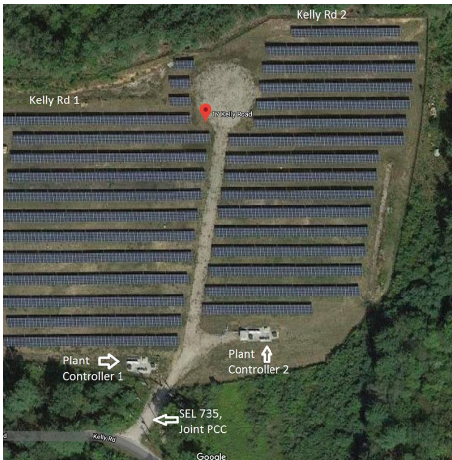
Figure 2. Satellite Photo of Kelly PV Plant #1 and #2
