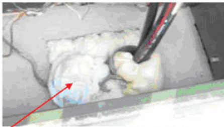
To seal spare conduit, install rag and fill with the expanding foam.
